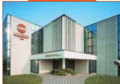
Plant n° 1 - Shrink division - DALMINE
